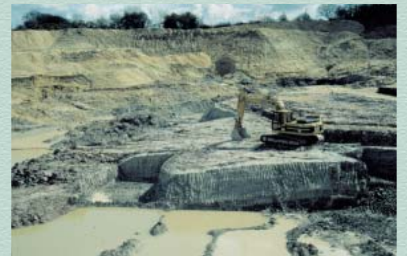
Doreys pit working Creekmoor Clay.
